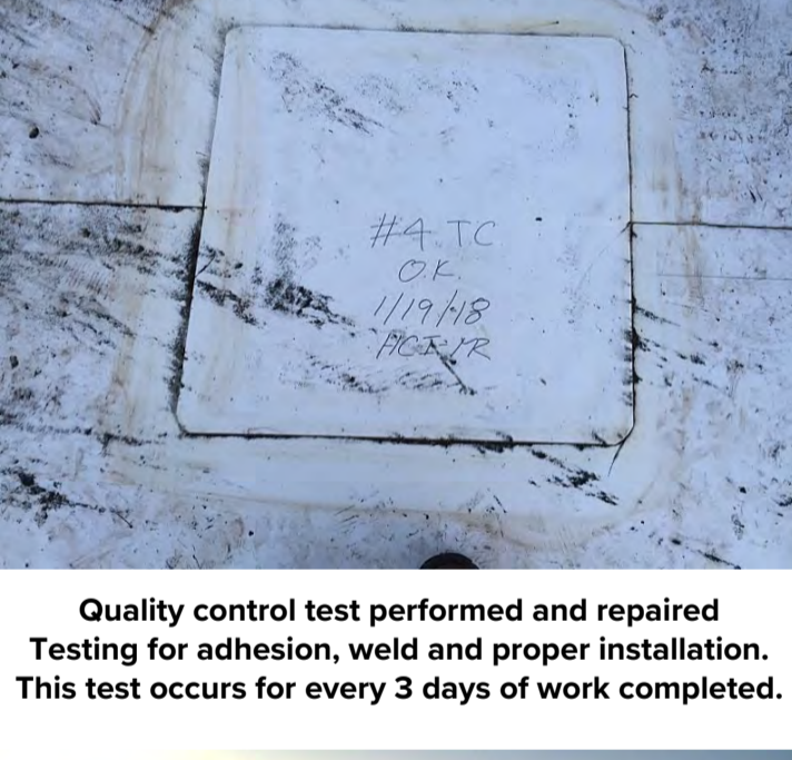
Plates installed by specs.
