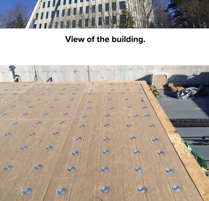
New deck mechanical fastener.
