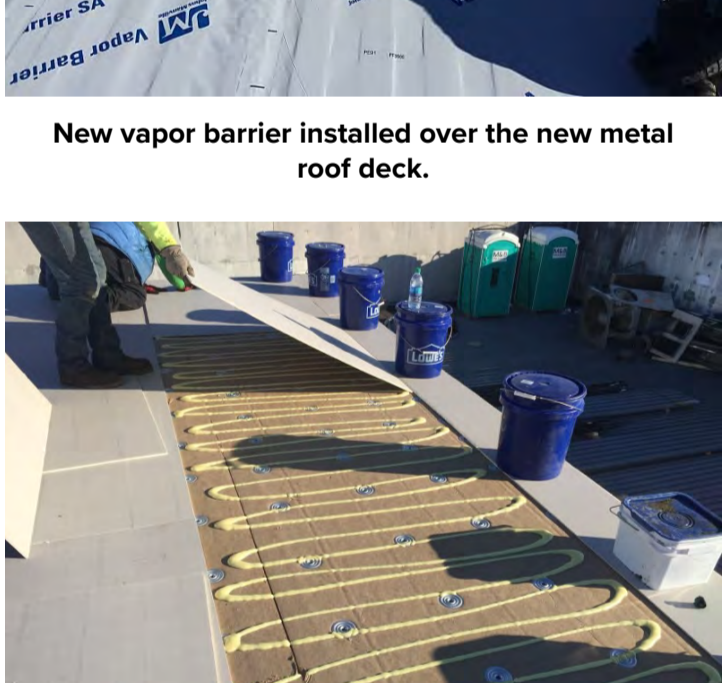
New insulation installation.
