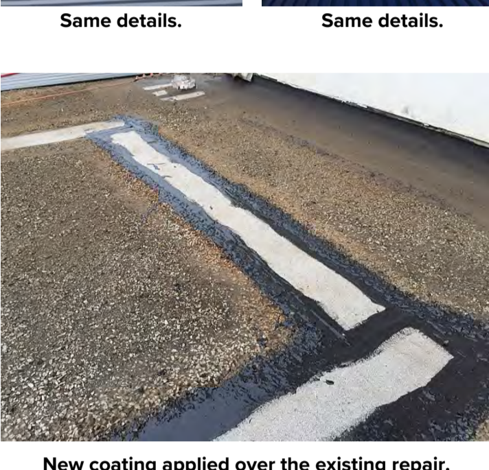
Temporary flashing in place with new base sheet.
